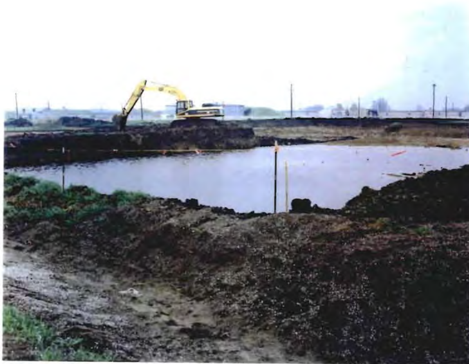
Photo No. 7: (30 April 1997) Excavation of contaminated materials as viewed looking northwest.
