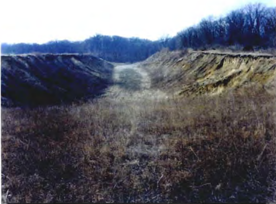
Photo No. 1: (12-16 March 1996) Preconstruction conditions along Trench 6, looking south.
