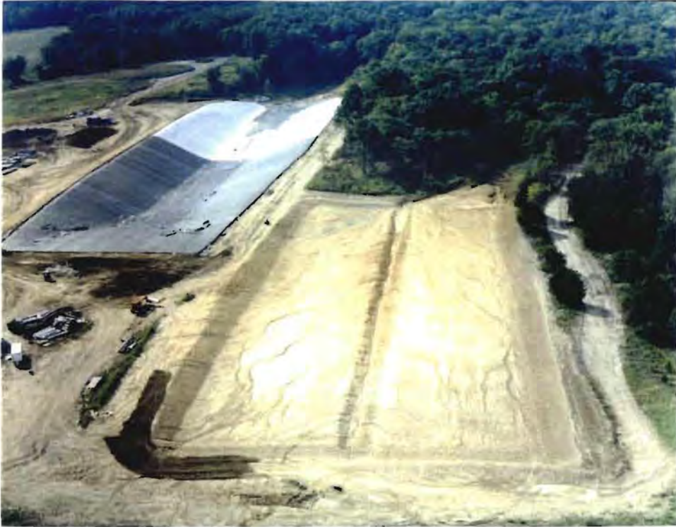
Photo No. 3: (17-18 September 1996) Aerial view of the CAMU and Trench 6.
