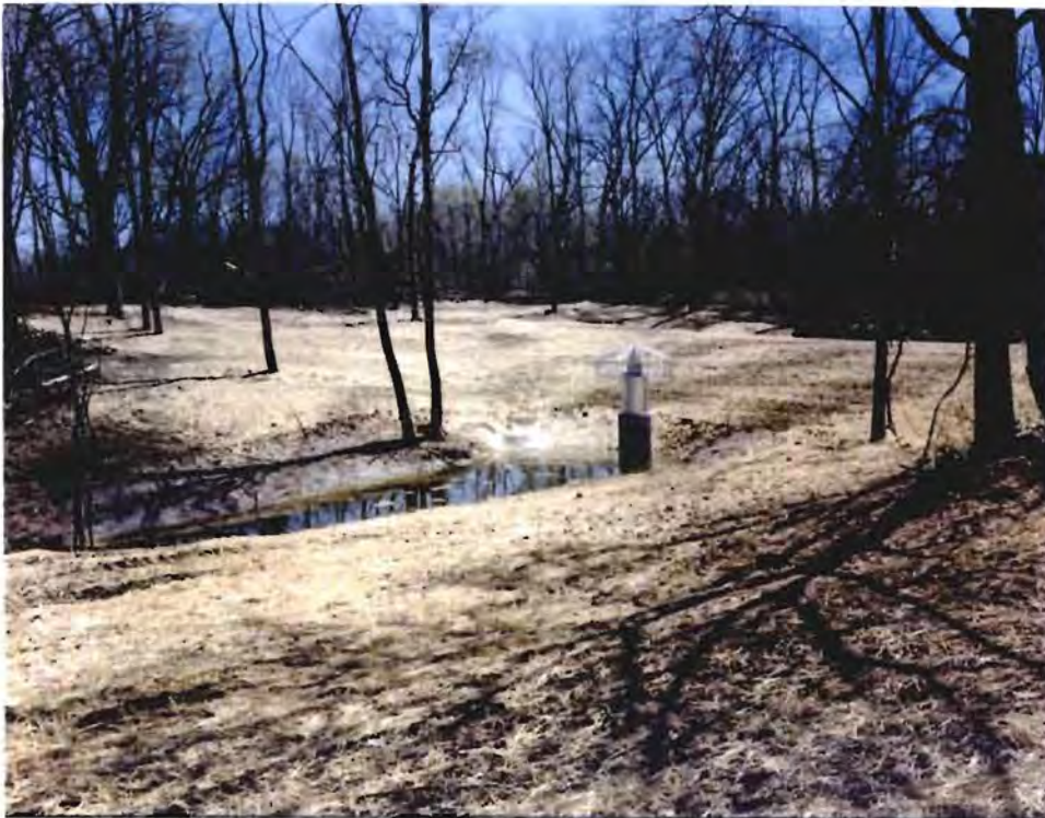
Photo No. 6: (1 May 1997) View of the completed Sediment Dam. Note the riser which was added to the intake structure to prevent the uncontrolled release of contaminated water from the CAMU site.
