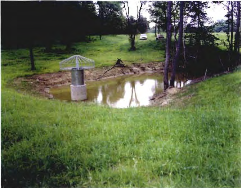
Photo No. 7: (24 June 1997) View of the completed Sediment Dam.
