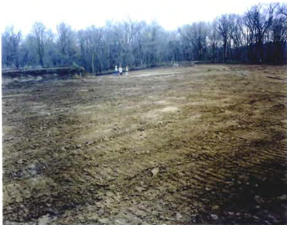
Photo No. 2: (1 May 1997) View of the remediated Explosives Sumps Stockpile and the Burning Grounds looking southwest. The Explosives Sumps Stockpile was placed into the Trench 6 Soils Repository.
