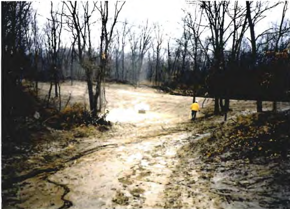
Photo No. 5: (March 1997) View of the completed Sediment Dam. Note that the water elevation behind the dam is near the invert of the uncontrolled intake structure.
