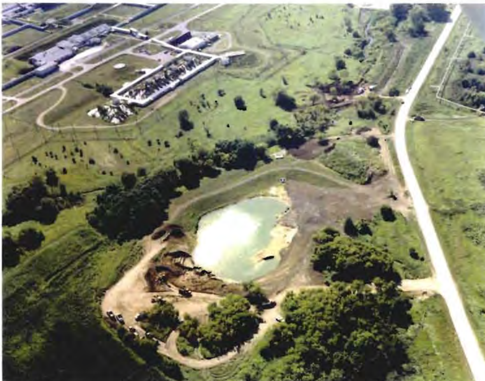
Photo No. 10: (7 August 1997) Aerial view of the complete Wetland Borrow Area Dam. Borrow excavation is continuing in the upstream reaches of the reservoir.
