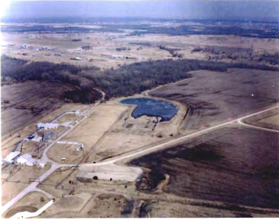
Photo No. 1: (12-16 March 1996) Preconstruction aerial view of the Line 800 Pinkwater Lagoon looking northwest.
