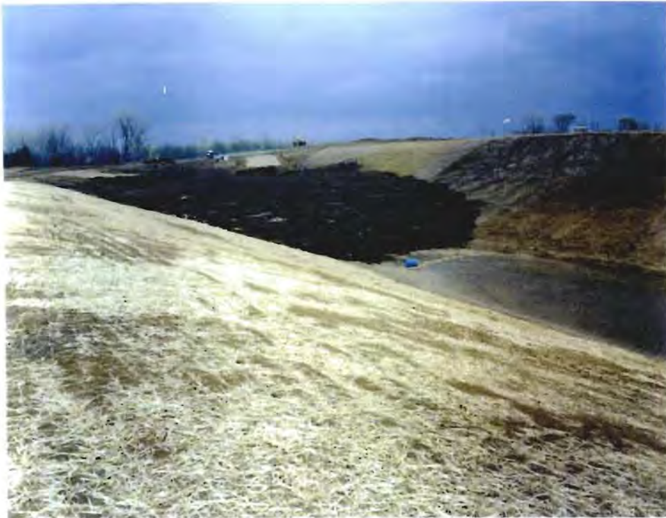
Photo No. 14: (1 May 1997) View of the north end of Trench 6 where contaminated soil from the Line 1 Impoundment and the Line 800 Lagoon has been placed.
