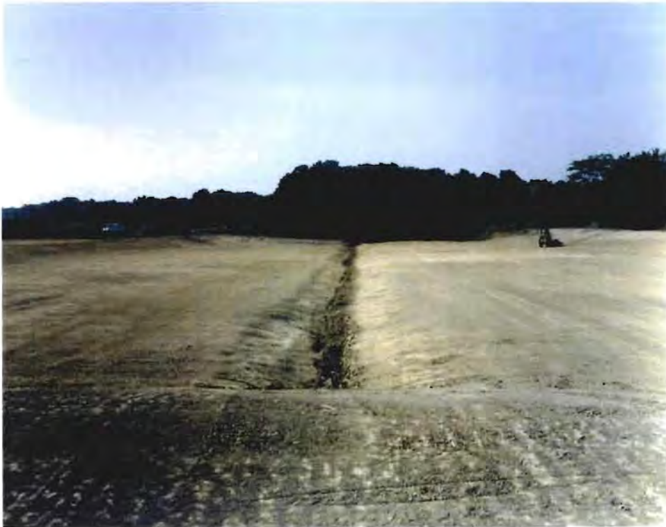
Photo No. 2: (15 August 1996) Initial grading of the CAMU, looking south.
