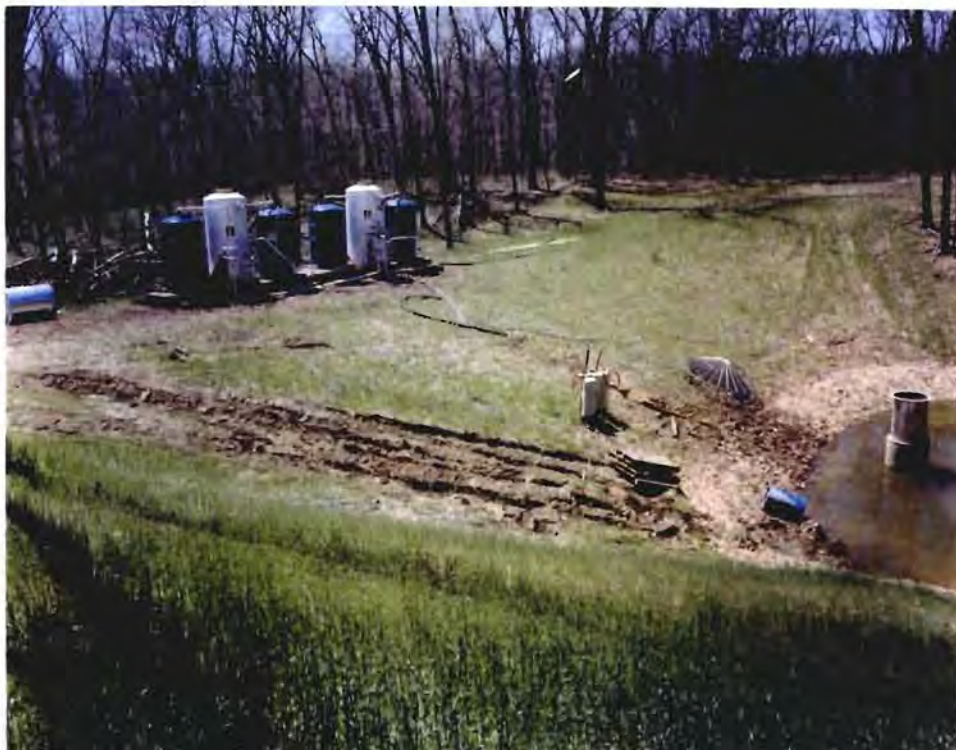
Photo No. 10: (1 May 1997) View of the granular activated carbon (GAC) units located on top of the embankment. The GAC units are used to treat the contaminated storm water and leachate from the Inert Disposal Area prior to releasing to the downstream channel. When construction of the landfill cap is completed, and the subsequent inflow of contaminated water into the Sediment Dam ceases, the GAC units will be disassembled and inflows will be released through the uncontrolled outlet works.
