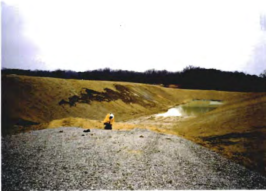
Photo No. 13: (March 1997) View of Trench 6 after the protective soil cover had been placed. The soil repository had just begun to receive contaminated materials. A slide of the cover soil had occurred on the east sideslope of the trench at the geogrid/soil interface. There was no damage to any of the geosynthetic layers.
