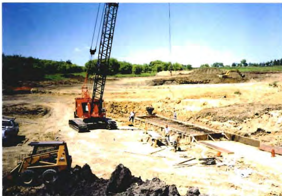
Photo No. 3: (8 August 1996) Construction of the outlet works conduit in progress.
