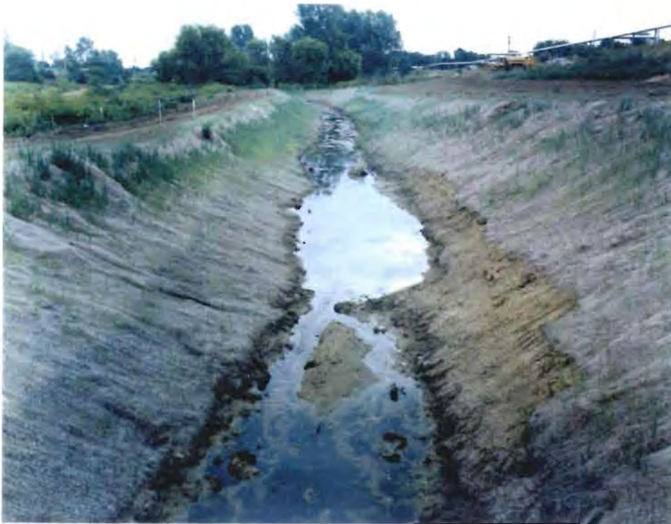
Photo No. 8: (15-16 July 1996) View of the relocated Brush Creek flowing southeast (downstream) around the Line 1 Impoundment as viewed from the temporary construction crossing.
