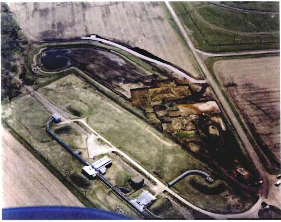
Photo No. 6: (1 May 1997) Aerial of the excavation of contaminated materials as viewed looking easterly.
