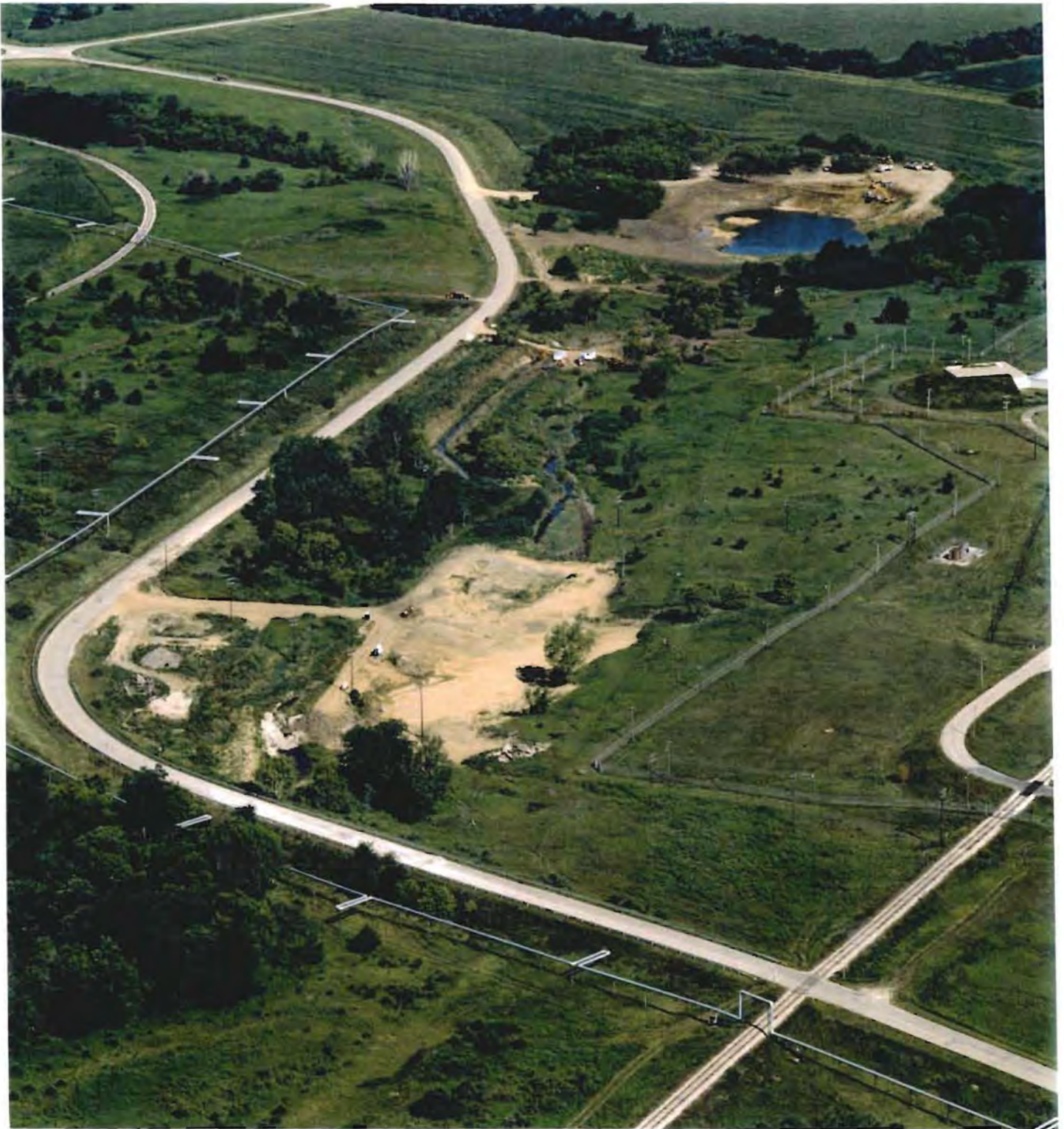
Photo No. 4: (7 August 1997) Aerial photograph of the Line 1 Impoundment as viewed looking northwest. Construction is in progress of the upstream wetland hydraulic control structure. Material is still being mined from the Wetlands Borrow Area.
