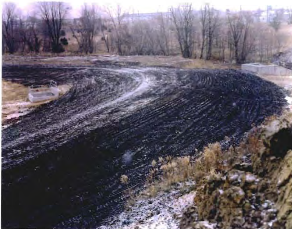
Photo No. 8: (19 November 1996) The Wetland Borrow Area embankment is complete.
