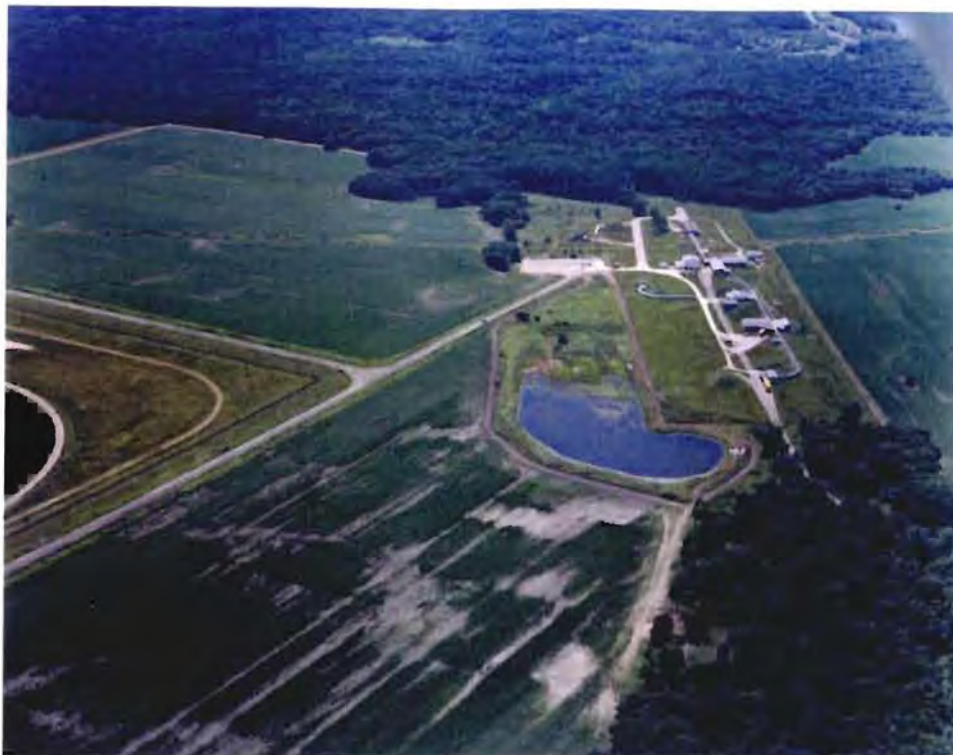
Photo No. 3: (15-16 July 1996) Aerial view of the Line 800 Pinkwater Lagoon looking southeast. Note the granular activated carbon units on the embankment crest. The lagoon is being dewatered.
