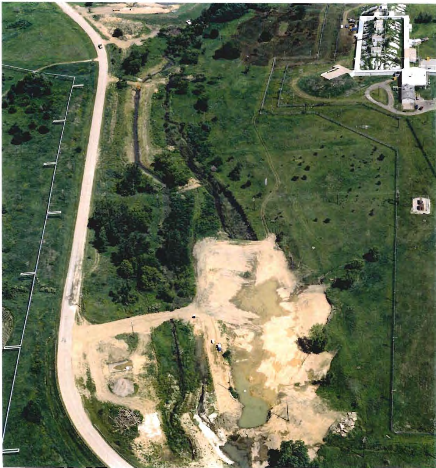
Photo No. 3: (24 June 1997) Aerial photograph of the Line 1 Impoundment as viewed looking northwest. 8,270 cubic yards of contaminated soil containing 3,937 pounds of explosives has been excavated and relocated to the Inert Disposal Area.
