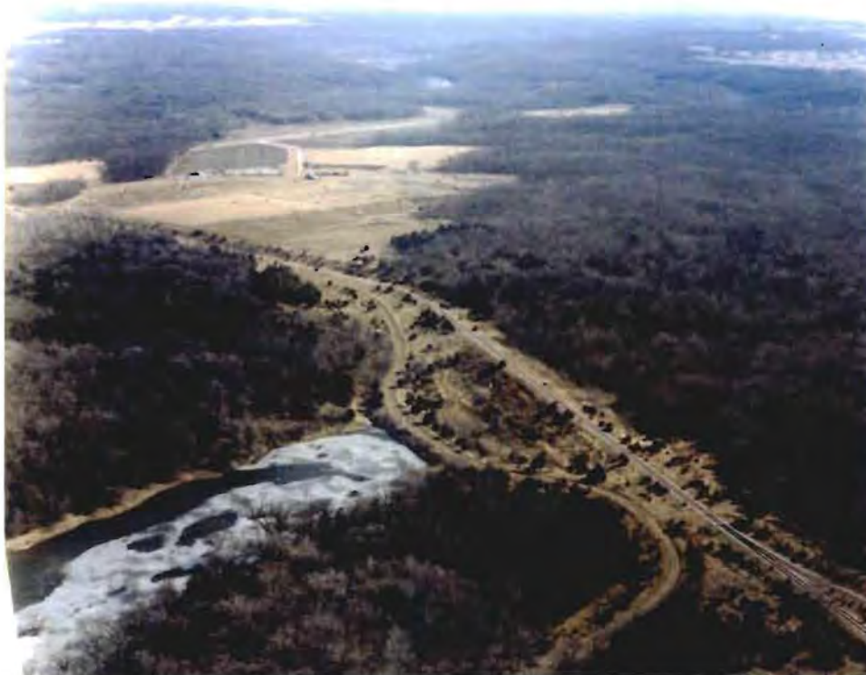
Photo No. 1: (12-13 March 1996) Aerial view of the original Stump Lake and Dam prior to breaching of the dam. Note the Inert Disposal Area in the background.
