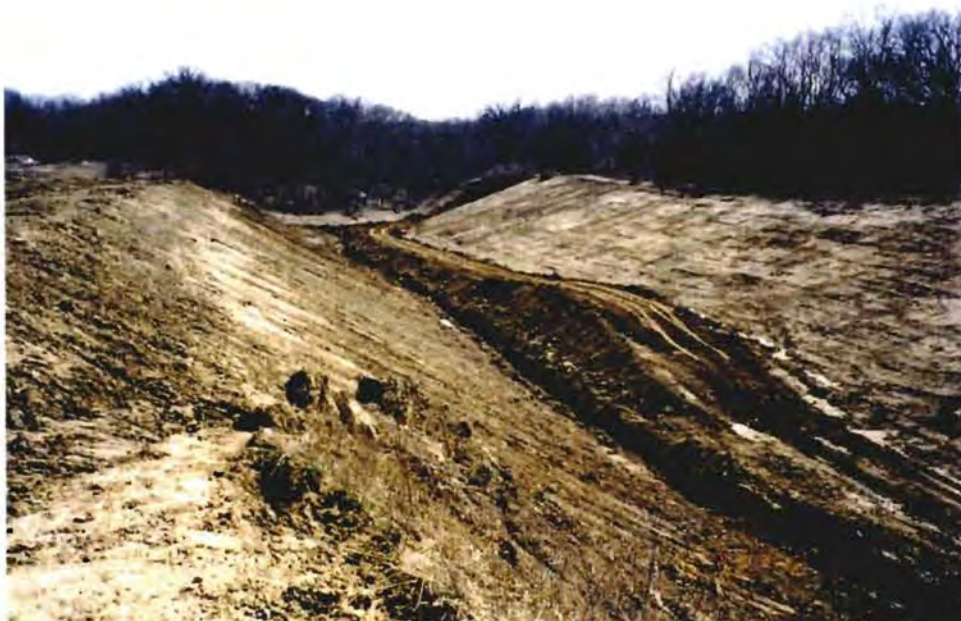
Photo No. 2: (March 1996) Initial grading of Trench 6, looking south.
