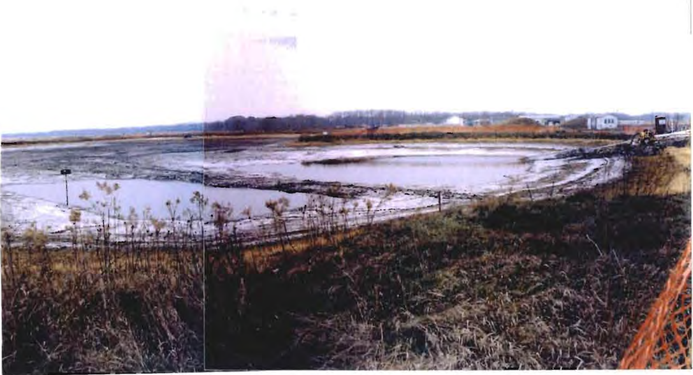
Photo No. 5: (19 November 1996) The Line 800 Lagoon has been essentially dewatered.
