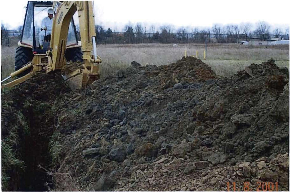
Photo #3: Fire Training Pit, Exploratory Trench FTA-T1, 8 November 2001 "Fuel-Contaminated Soil" Area Discolored (Greenish) Soil Visible in Excavated Soil
