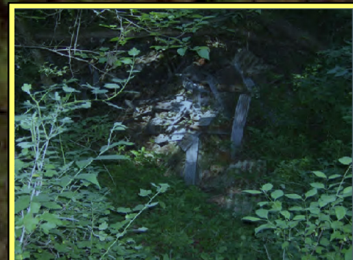
ACM Debris Pile located centrally within CC-IAAP-002 (looking east from ACM3)
