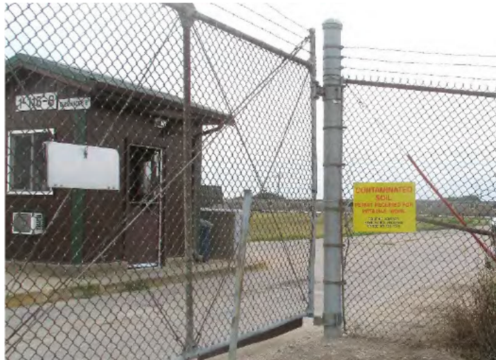
OU1 SIGN AT LINE 1 EAST ENTRANCE
