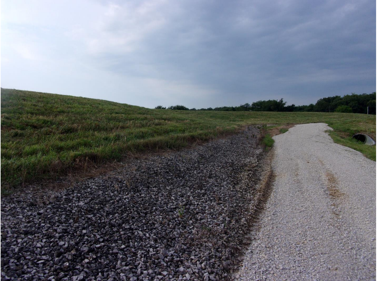
CEA west side looking south (August 2021).
