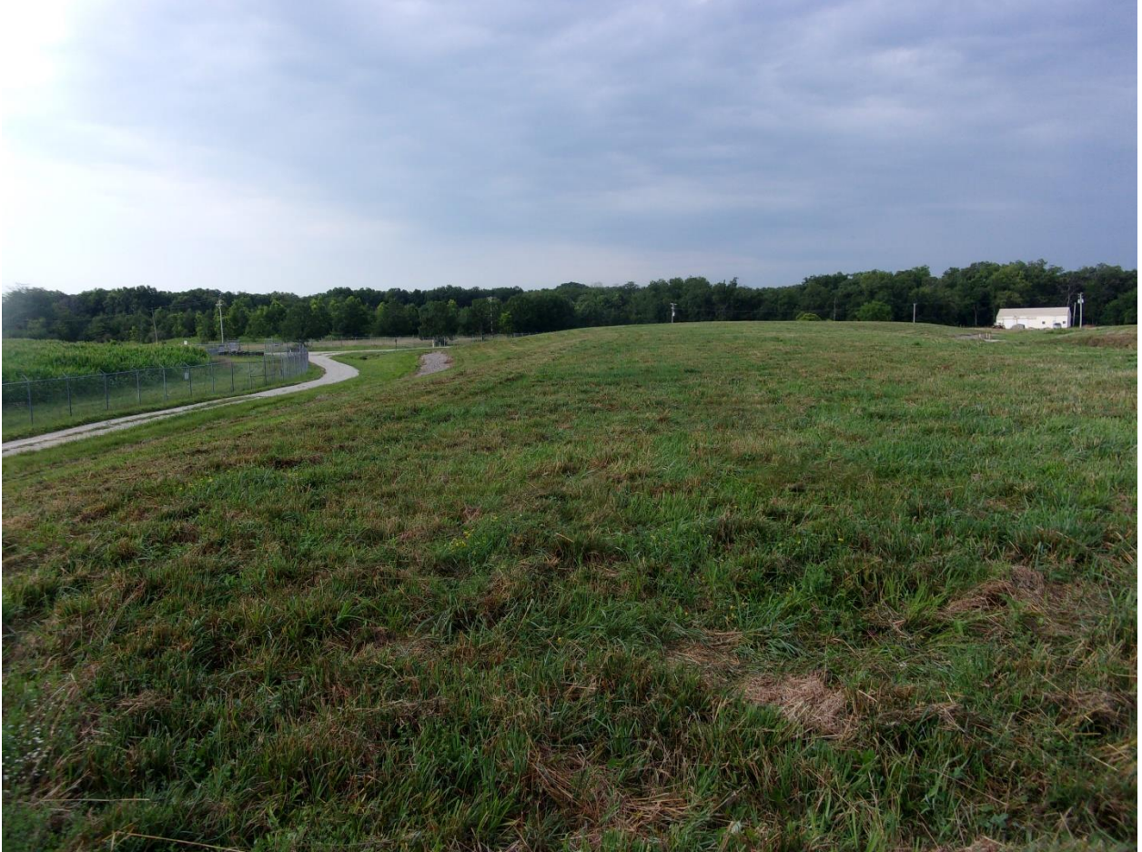
CEA North enc top looking south (August 2021).
