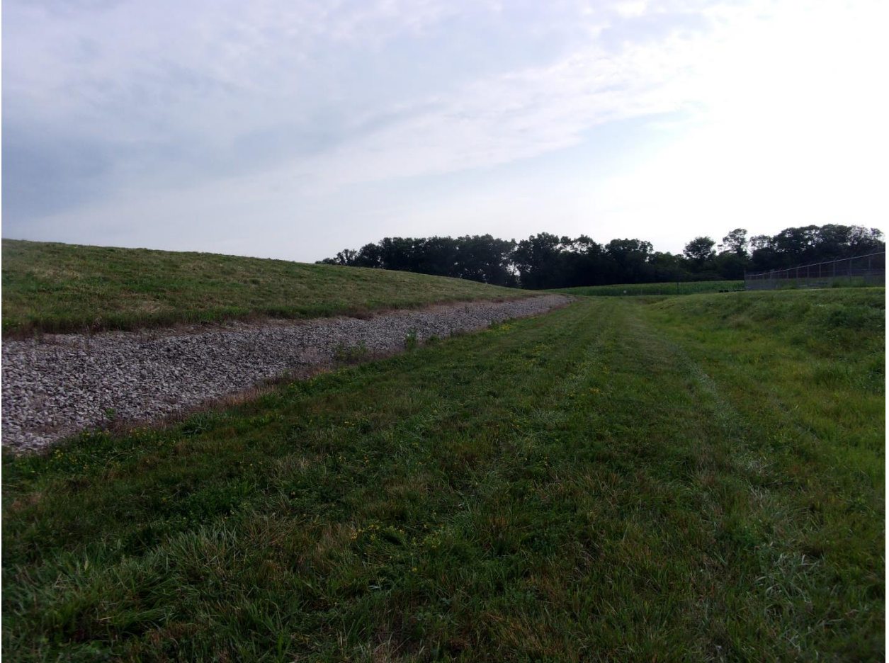
CEA toe drain east side looking north (August 2021).
