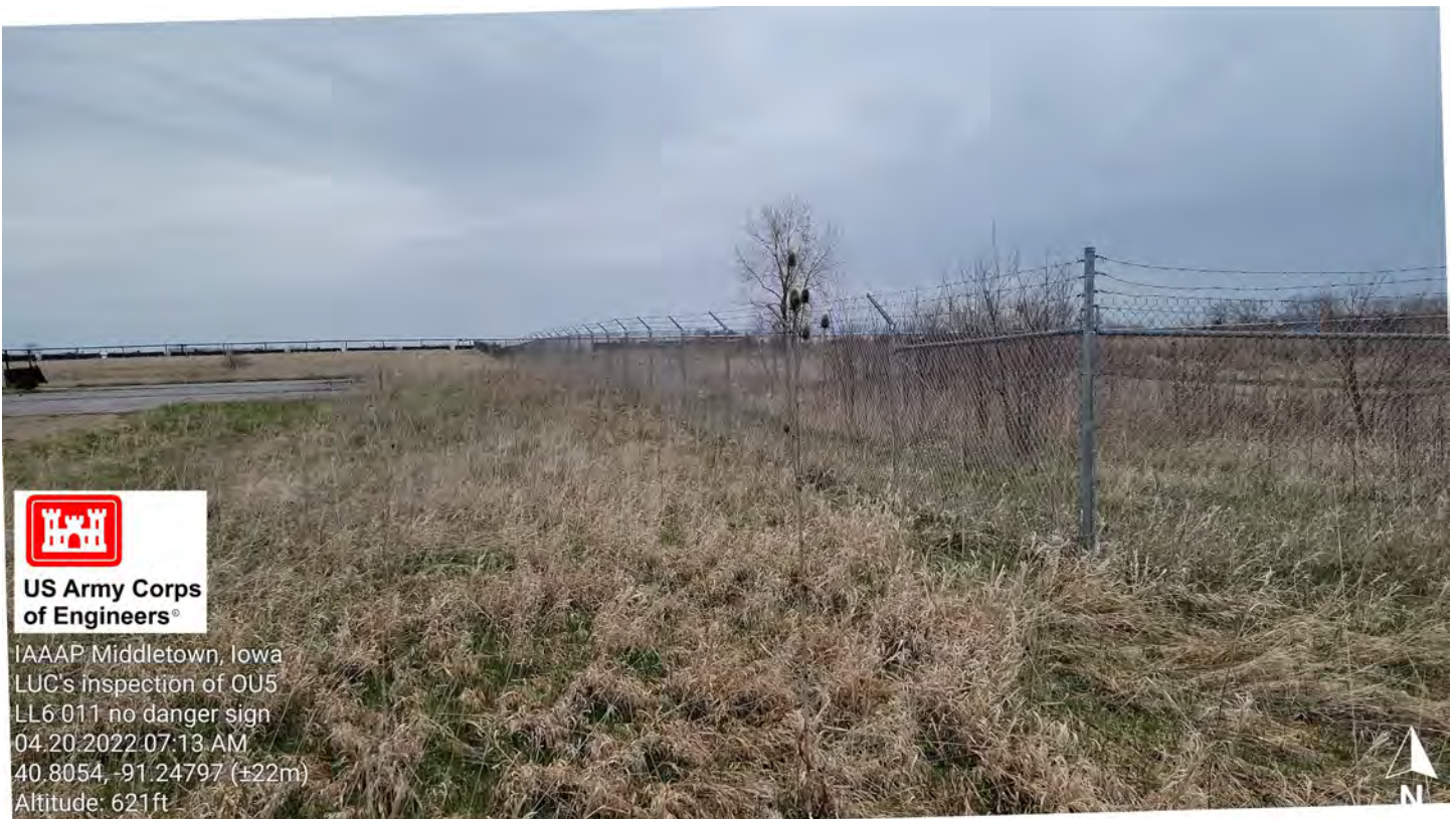
Photo 11 – LL6, Missing UXO Danger Sign
