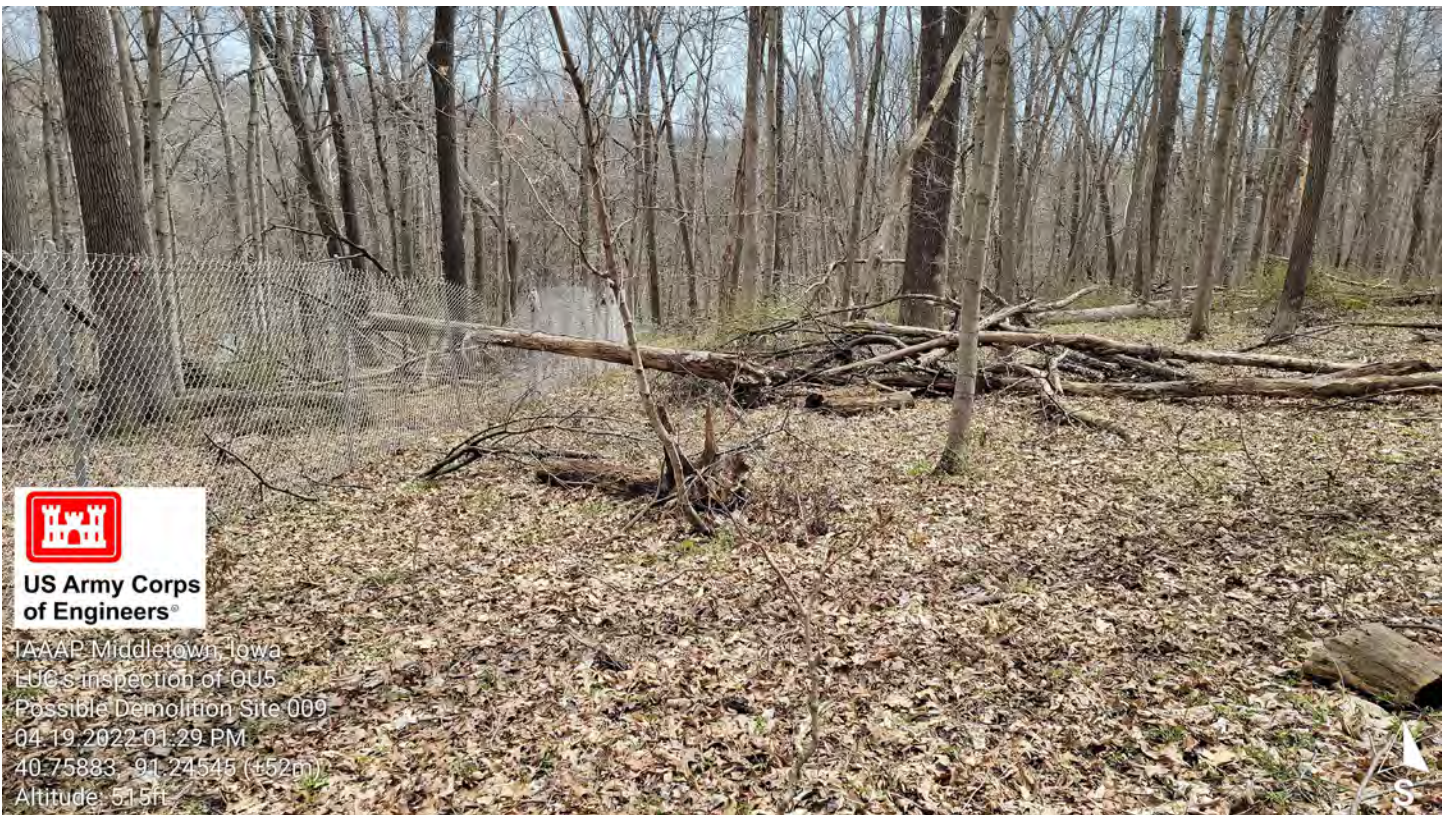
Photo 9– PDS, Approximately 10 feet damaged fence
