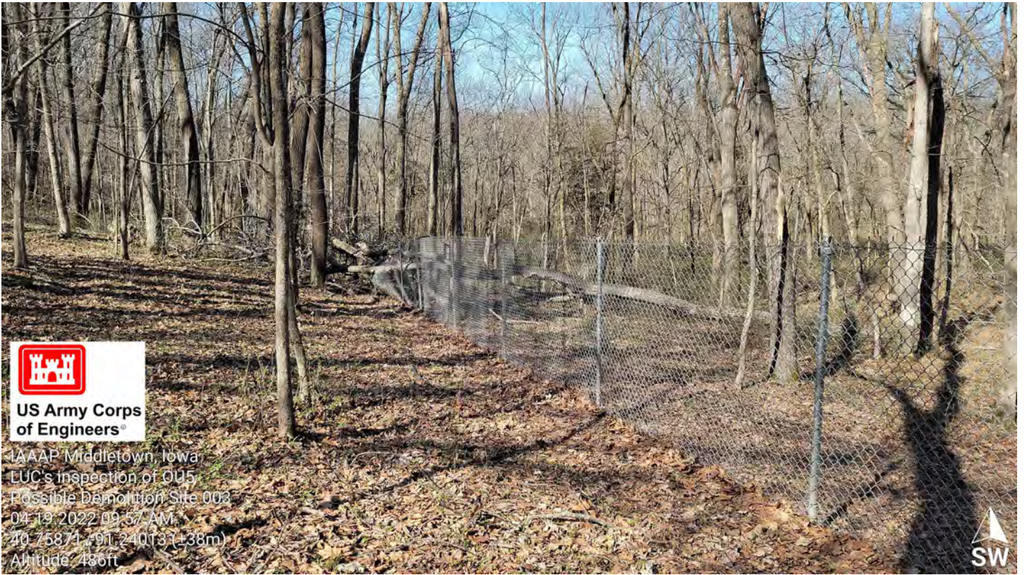
Photo 3 – PDS, Approximately 20 feet damaged fence.
