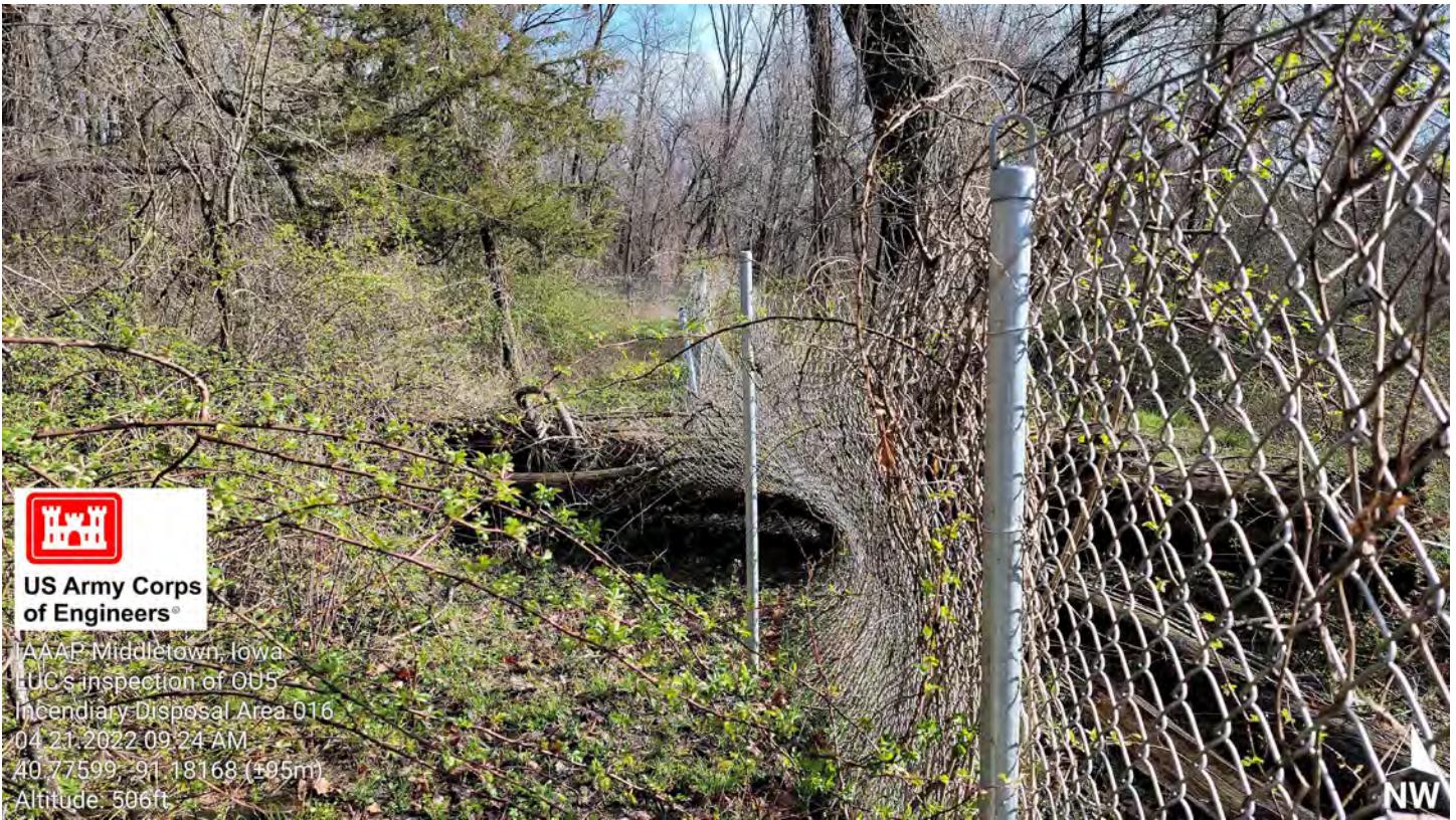
Photo 16 – InDA, 20 foot section of damaged fence.
