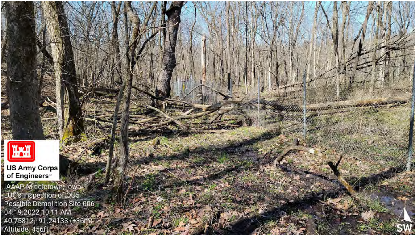
Photo 6 – PDS, Approximately 20 feet damaged fence.
