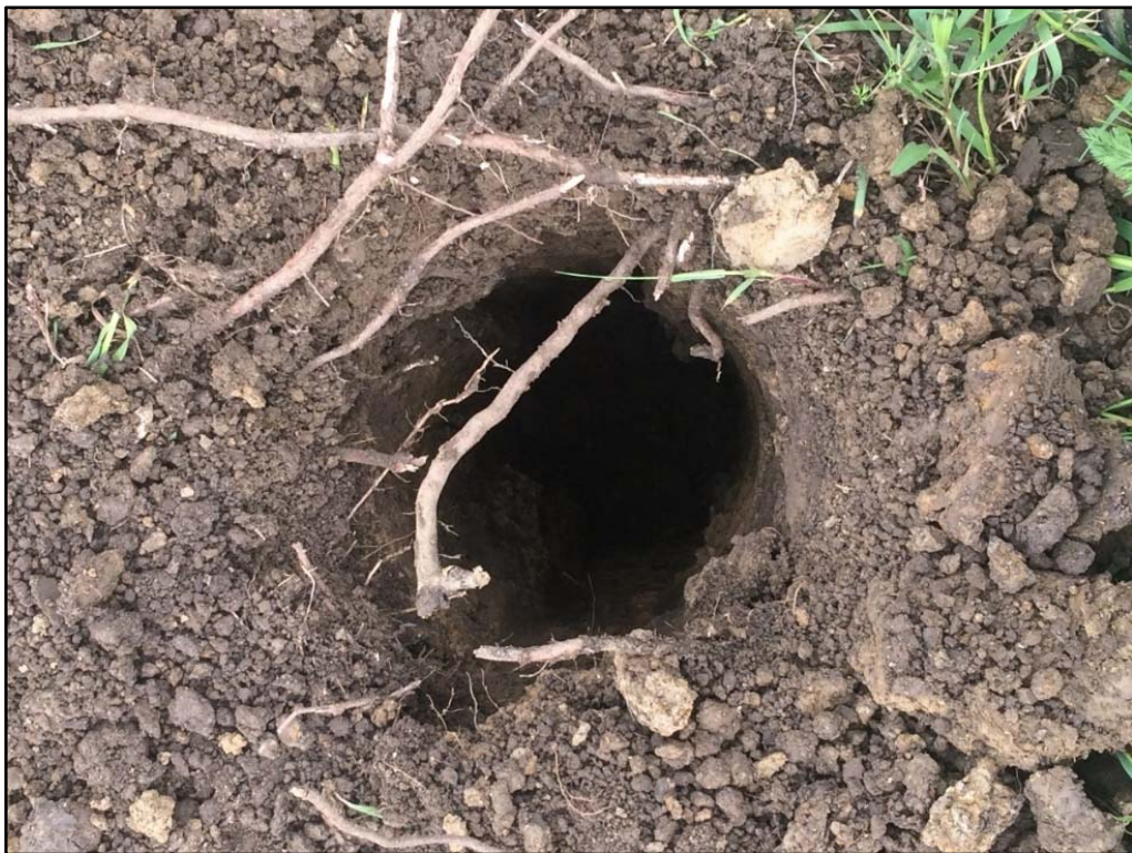
Photo 2. Ground view of a completed 12-inch fence post hole.
