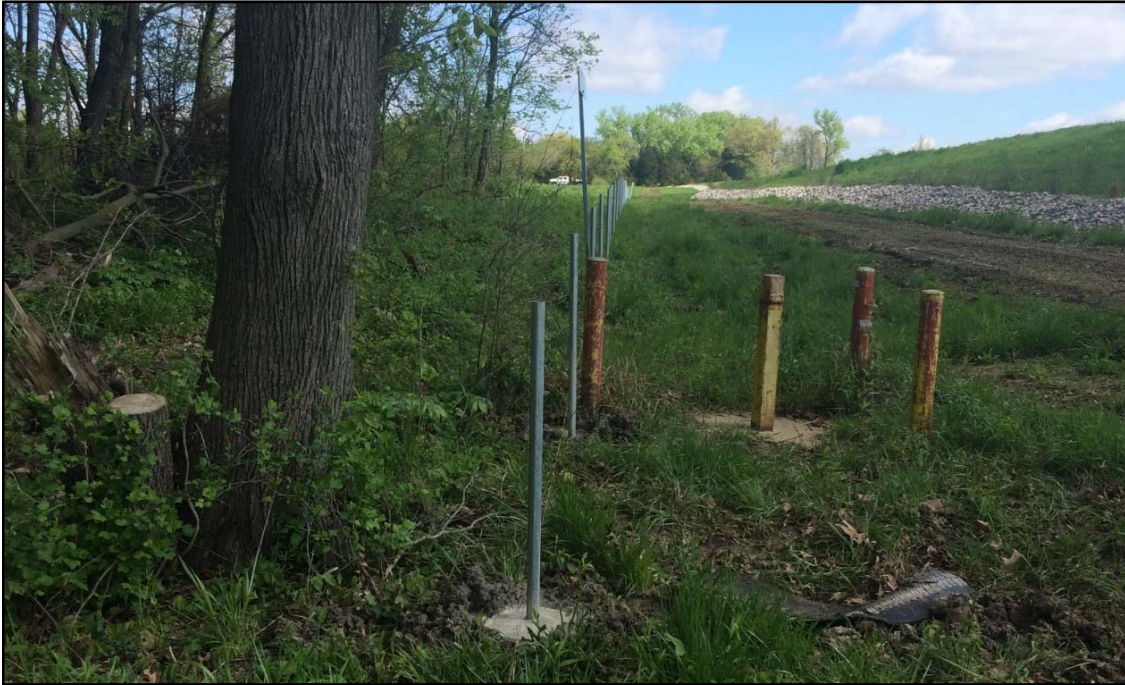
Photo 5. View north along the west side of Trench 6 Landfill. Showing fence posts secured in concrete.
