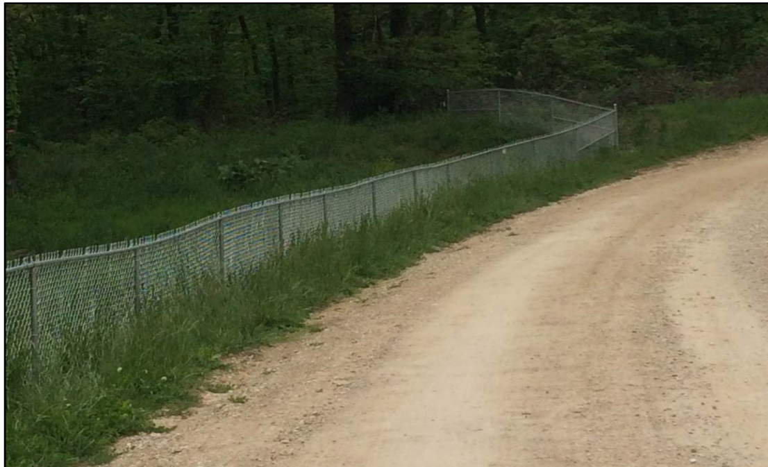
Photo 14. Showing where the newly constructed fence meets with the existing barbed wire fence that is the border of the active range.
